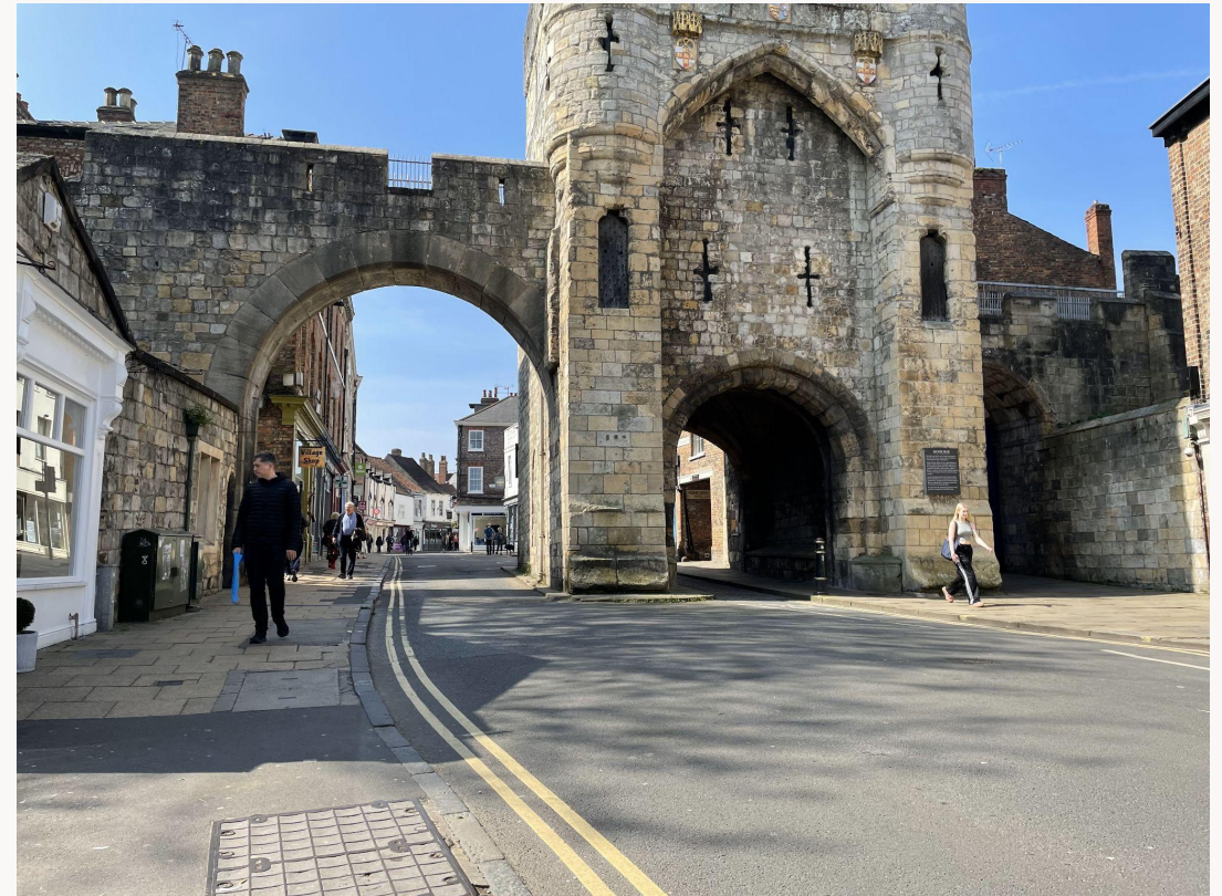
Photograph taken from Monkgate, looking towards Goodramgate and the City Walls.
